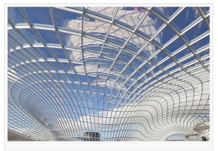
A striking 7000 square metre grid shell roof presents a milestone in structural design innovation as it arches over the atrium, soaring some 30 metres above the ground.
