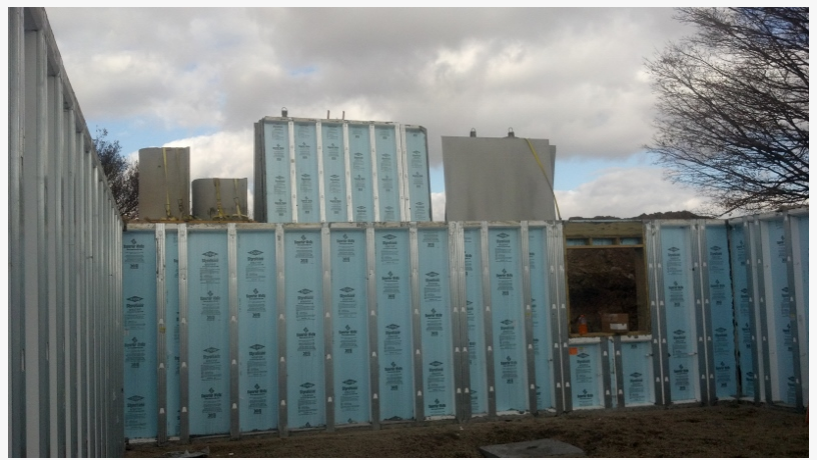
Superior Walls set as foundation for Legendary Homes project.
