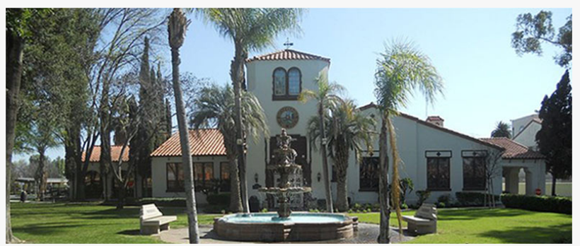
City of Perris, City Hall
