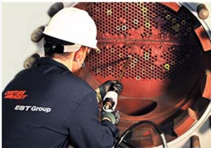
Installing a Pop-A-Plug®
